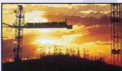
IN CIVIL WORKS
