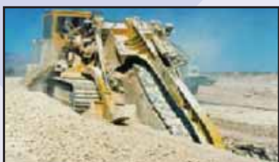
DURING LAYING AND DIGGING OPERATIONS
